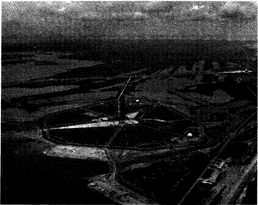
FIGURE D-18.—Launch complex 39D with vehicle 500 F in place.
