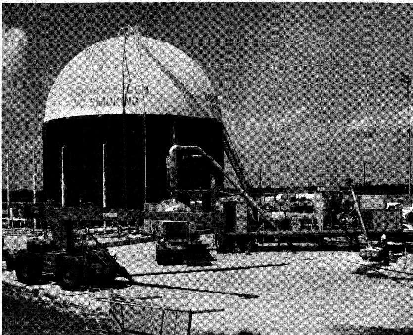
FIGURE D-19.—Liquid oxygen storage tank at launch complex 39, pad A.
